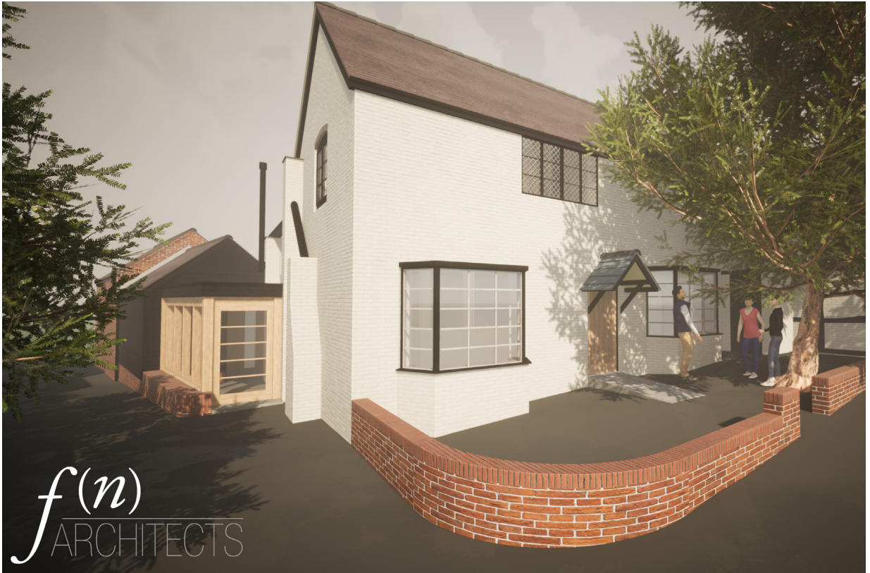
The view from Kitchen Hill Road showing the new toilet block.
